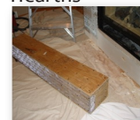
Wire Mesh applied over drywall.
