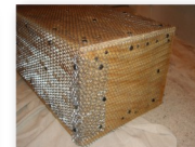
Scratch-coat of mortar applied.
